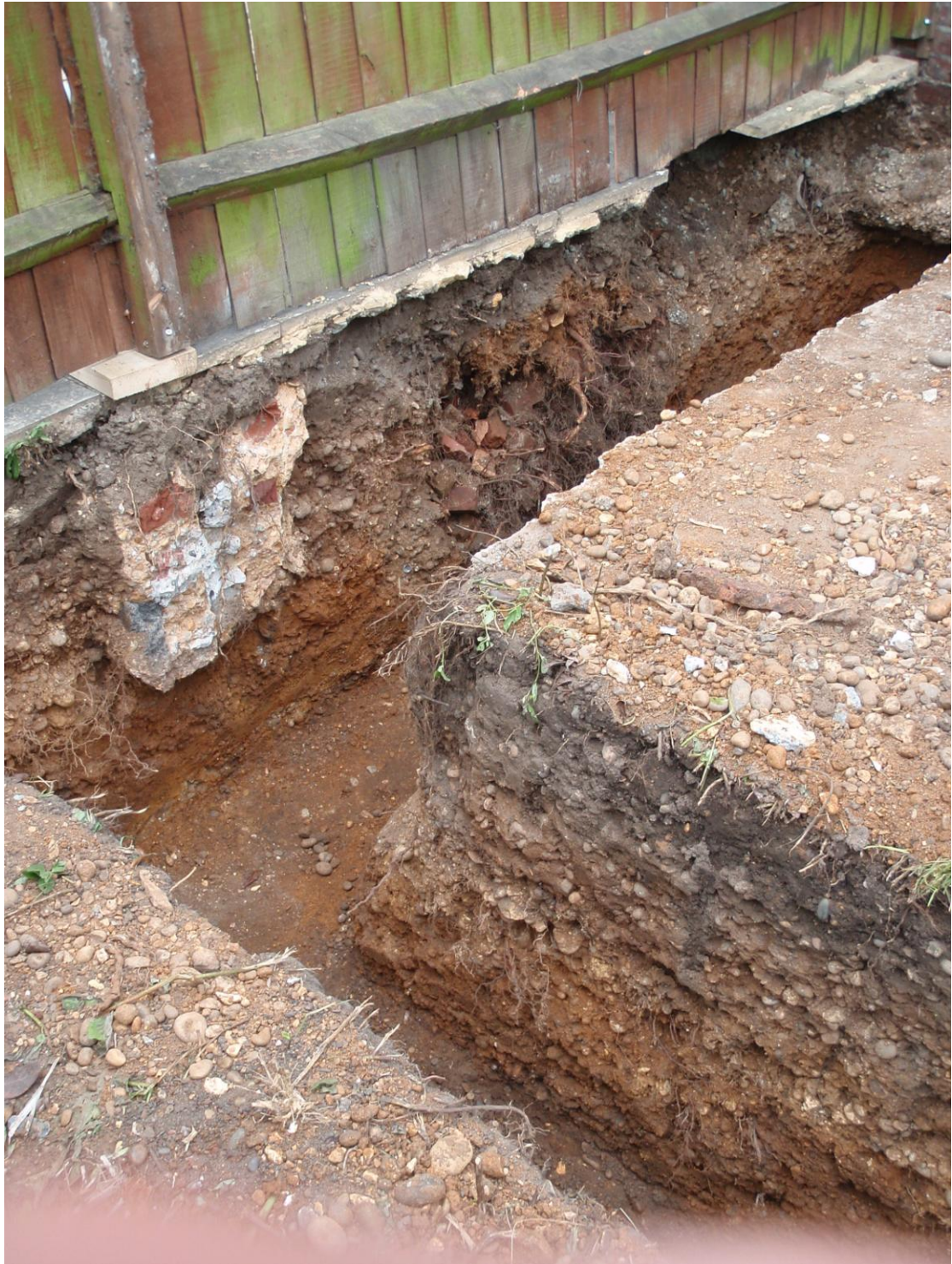
Plate 2. Showing previous modern impacts
